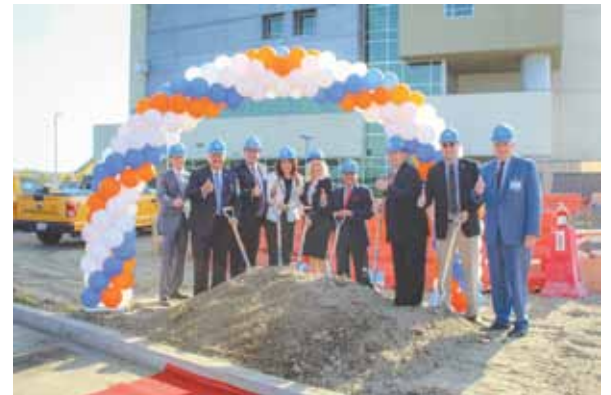
Kaiser Permanente Downey Medical Center broke ground on a new hospital tower, adding 96 beds and making the Downey campus Kaiser's second largest hospital in Southern California. The tower is scheduled to be completed by December 2020.
