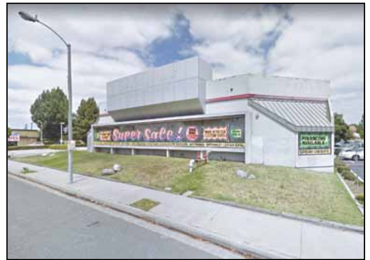
A proposed development at 18600 Gridley Road in Artesia would include 130 condominiums, a 20,000 sq. ft. restaurant, and retail shops.
