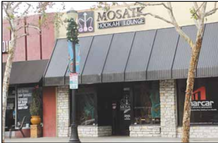
Excessive police calls and building violations prompted the Planning Commission to alter Mosaik Hookah Lounge's conditional use permit. Photo by Alex Dominguez
