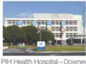
PIH Health Hospital – Downey
