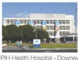
PIH Health Hospital - Downey
