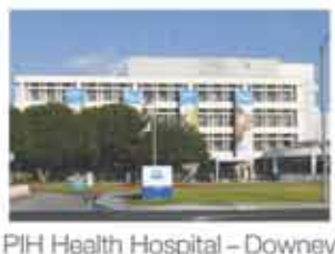
PIH Health Hospital – Downey
