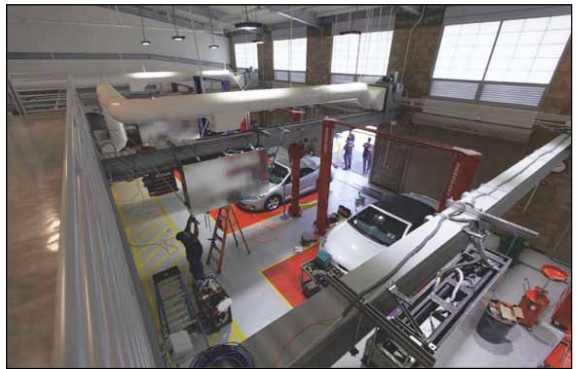
Downey High School's new engineering building, pictured above, will be open for a community open house next Thursday, Aug. 28, from 5:30-7:30 p.m., with official ceremonies at 6 p.m. Guests can tour the facility and get a first-hand look at some of the new technology being implemented in Downey schools.
