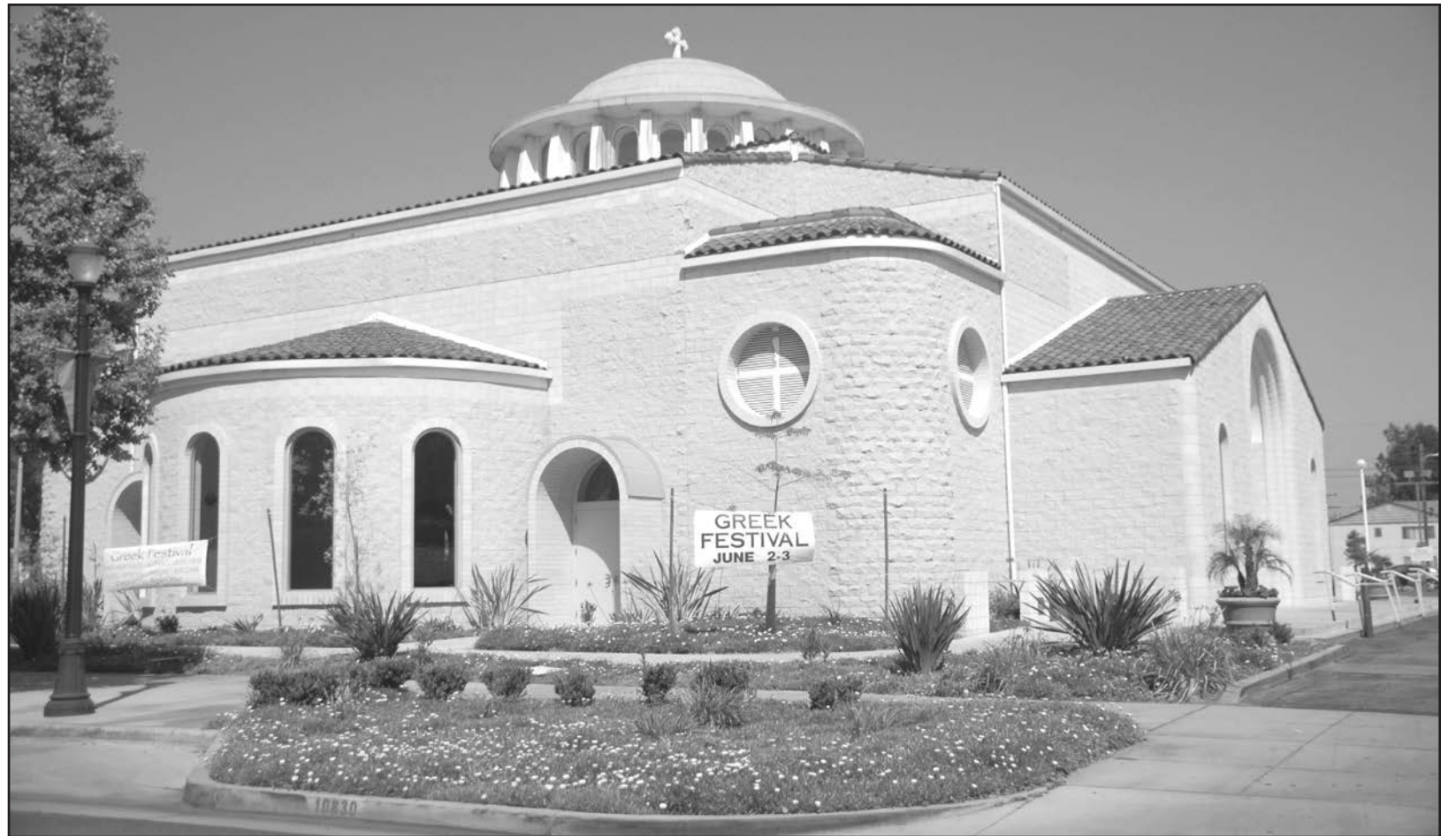
St. George Greek Orthodox Church sits on Downey Avenue. Its entrance faces south in anticipation of a future courtyard that will replace what is now Hi-Ho Market. Photo by Art Montoya
