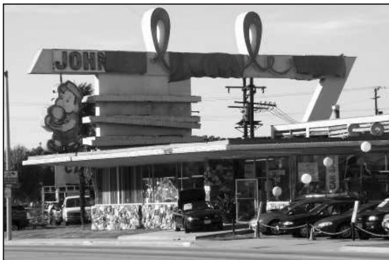
Blue tarps were draped over its signage when Johnie's Broiler was leased to a used car dealership in 2002. Photo courtesy Adriene Biondo
