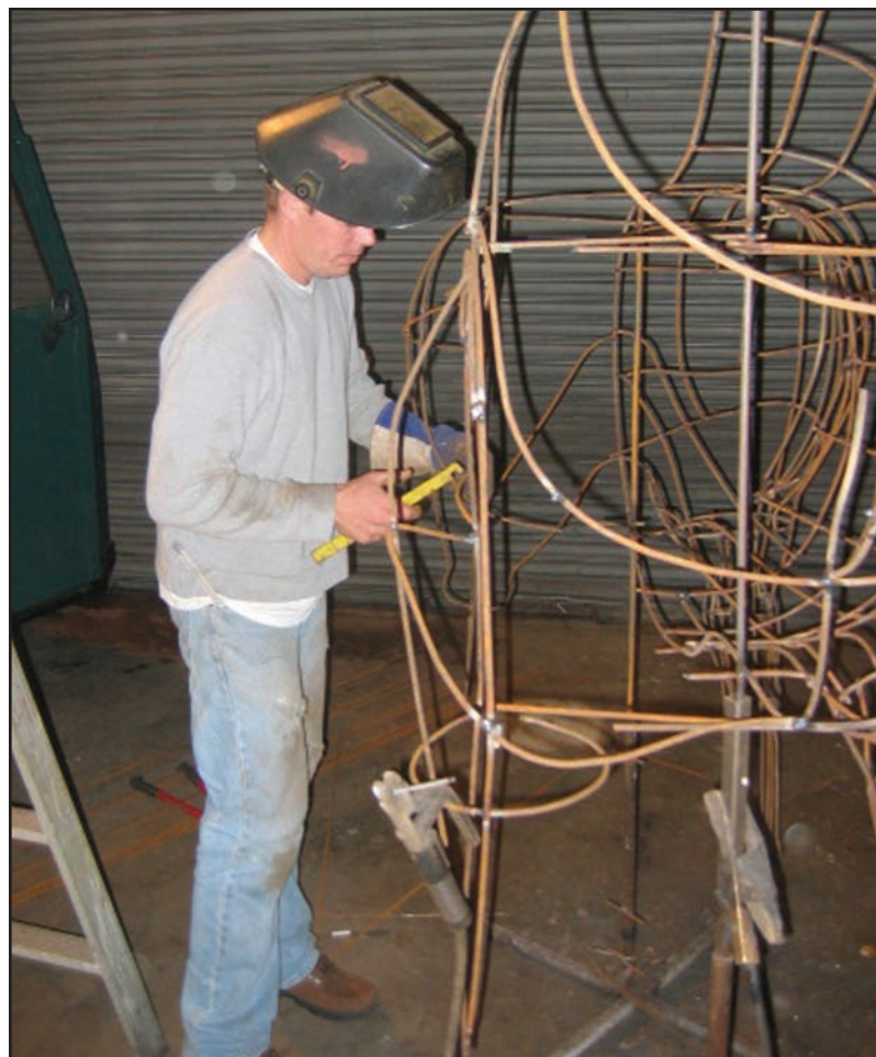
WELDING —A Rose Float volunteer was busy welding detail work on the float Tuesday. It will all be worthwhile when the big float appears as part of the Pasadena Rose Parade tomorrow.
